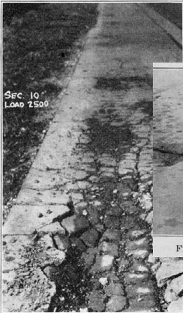
FIG. 11.—TYPICAL FAILURE OF ASPHALTIC CONCRETE SURFACING ON MACADAM BASE.
