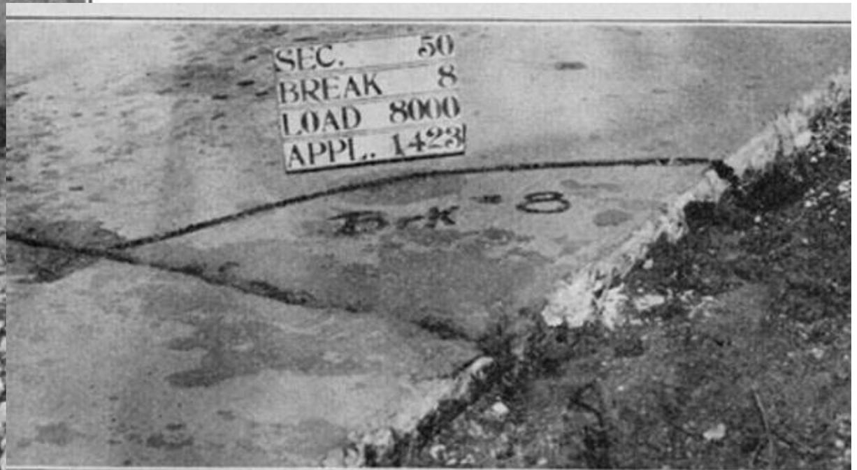
FIG. 18.—TYPICAL CORNER BREAK IN A CONCRETE SECTION.
