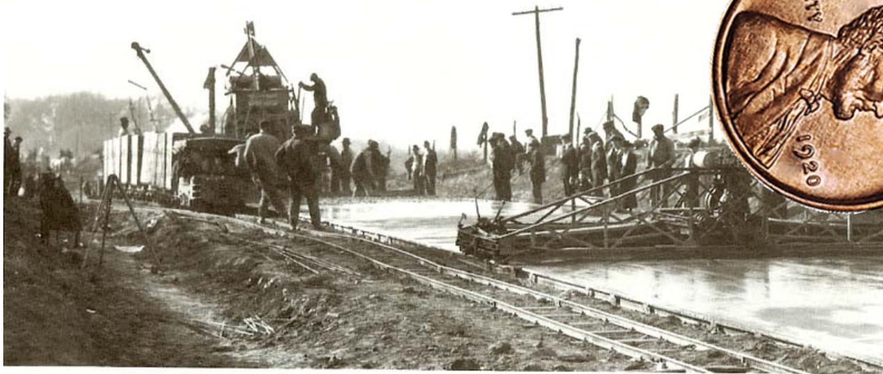
The leveling and smoothing machine follows the mixer, finishing the surface of new Highway 6.
