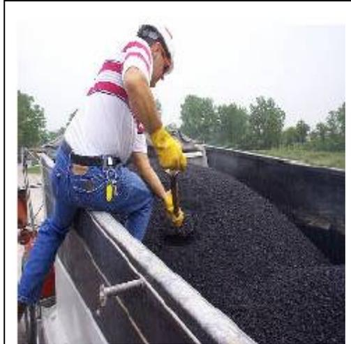
Figure 3. Sampling from haul units (After FHWA 1999).
