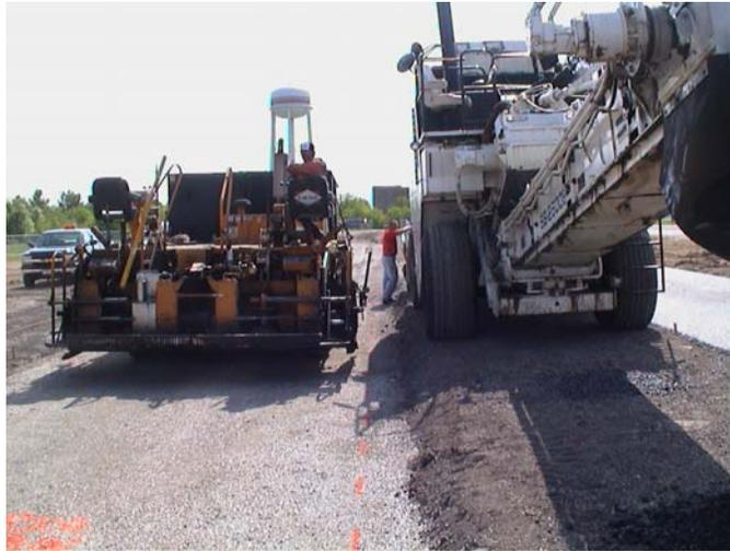
Figure 23. MTD on RAP center lane during paving.
