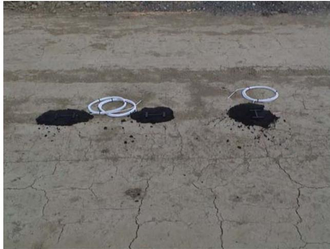
Figure 22. Placement of strain gauges.
