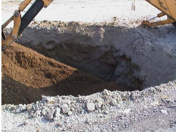
Figure 9. Excavation and replacement of soft grade and contaminated aggregate.
