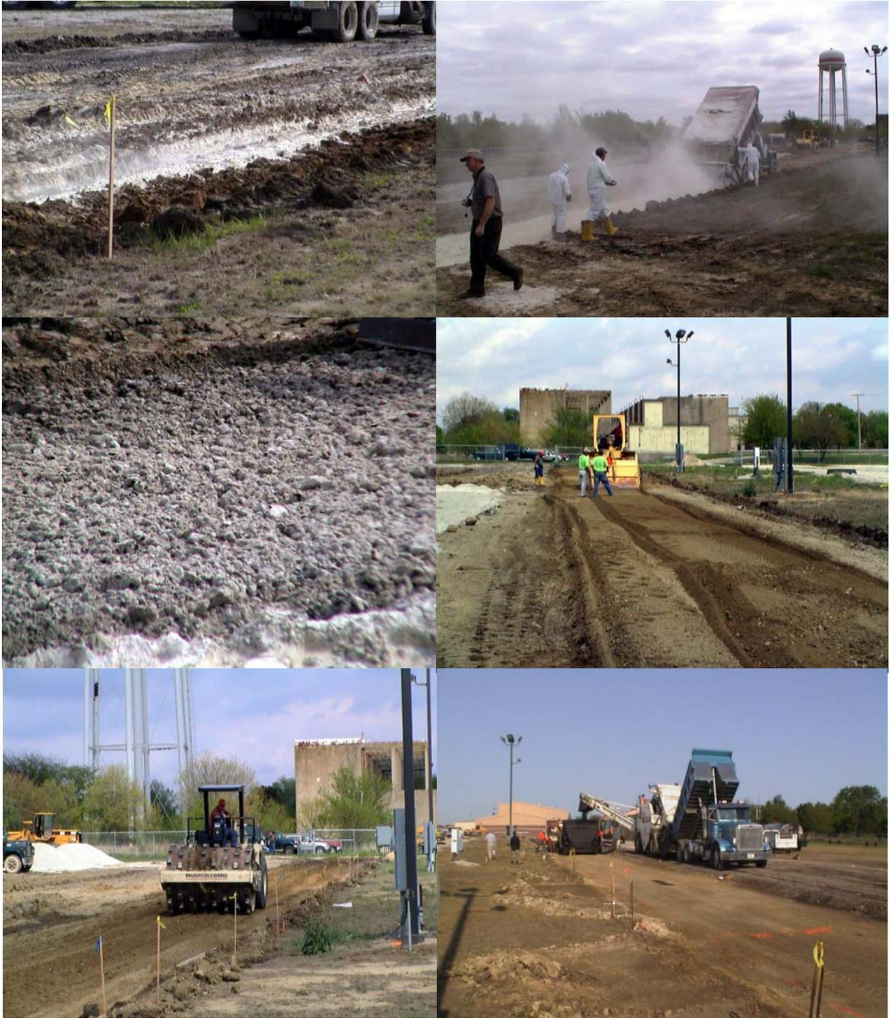
Figure 6. Construction of the lime-modified lane.
