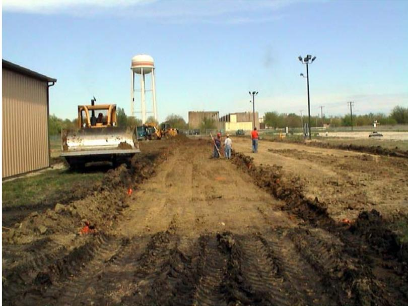
Figure 5. Lanes with topsoil removed.
