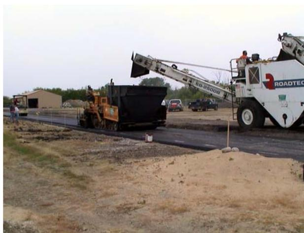
Figure 24. Paver and finish roller.
