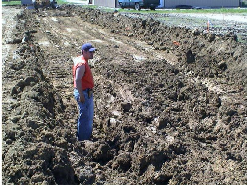
Figure 7. Undercutting at soft spot in Lane 1, aggregate lane.
