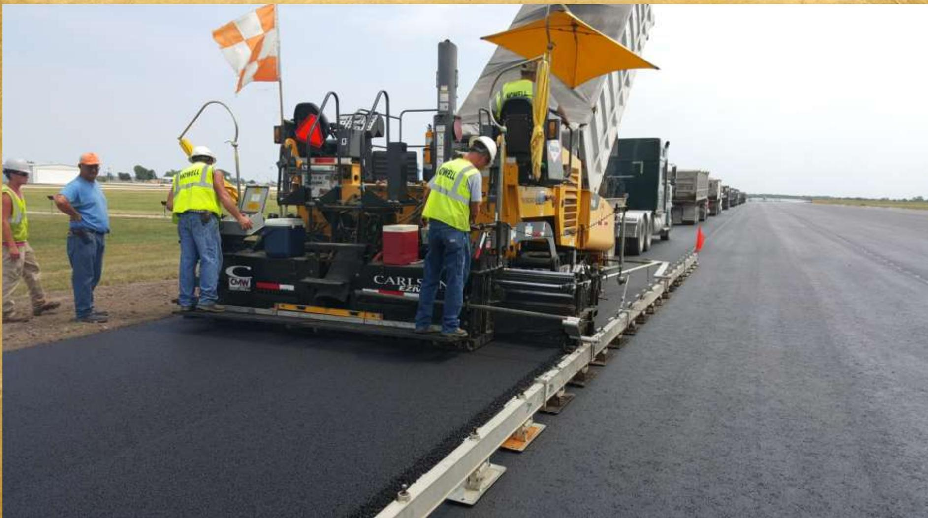
Except for First Pass 2-60' Skii's were used on Surface Mix (2" Lift Thickness)
