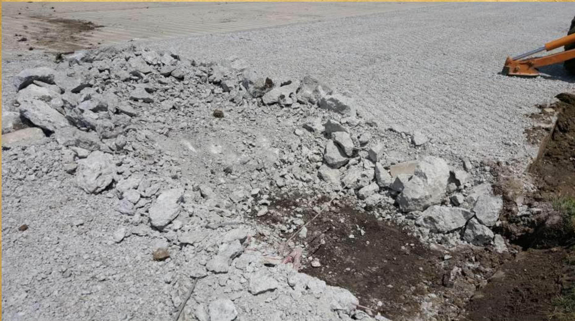
**Test Hole to ensure Complete Rubilization**
