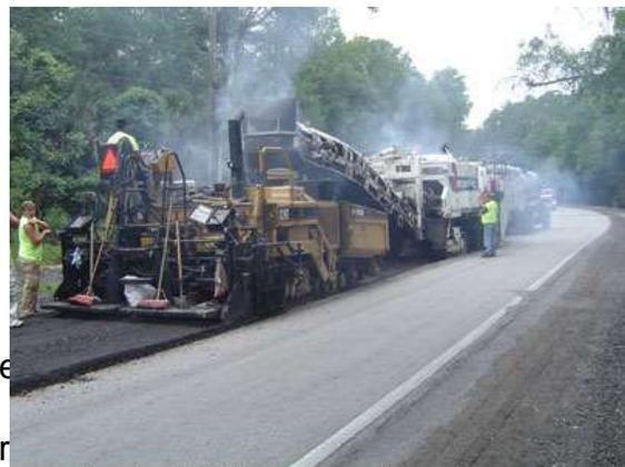
Fig. 2 - RAP being used in a hot mix
