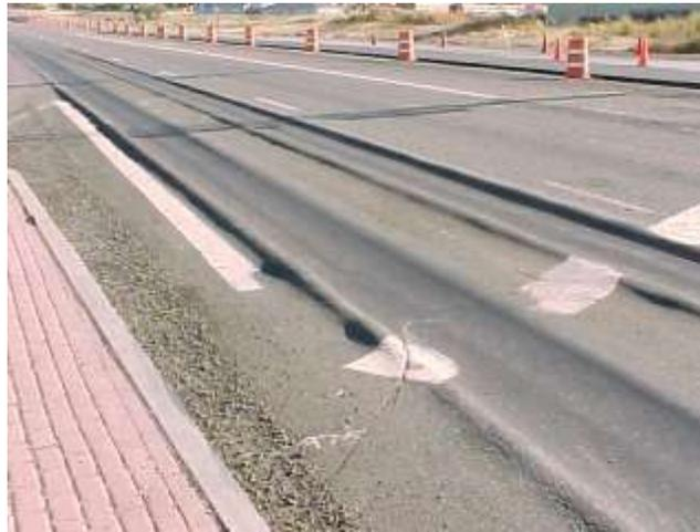
**Figure 1: Pavement Rutting (Pavement Interactive n.d.)**
