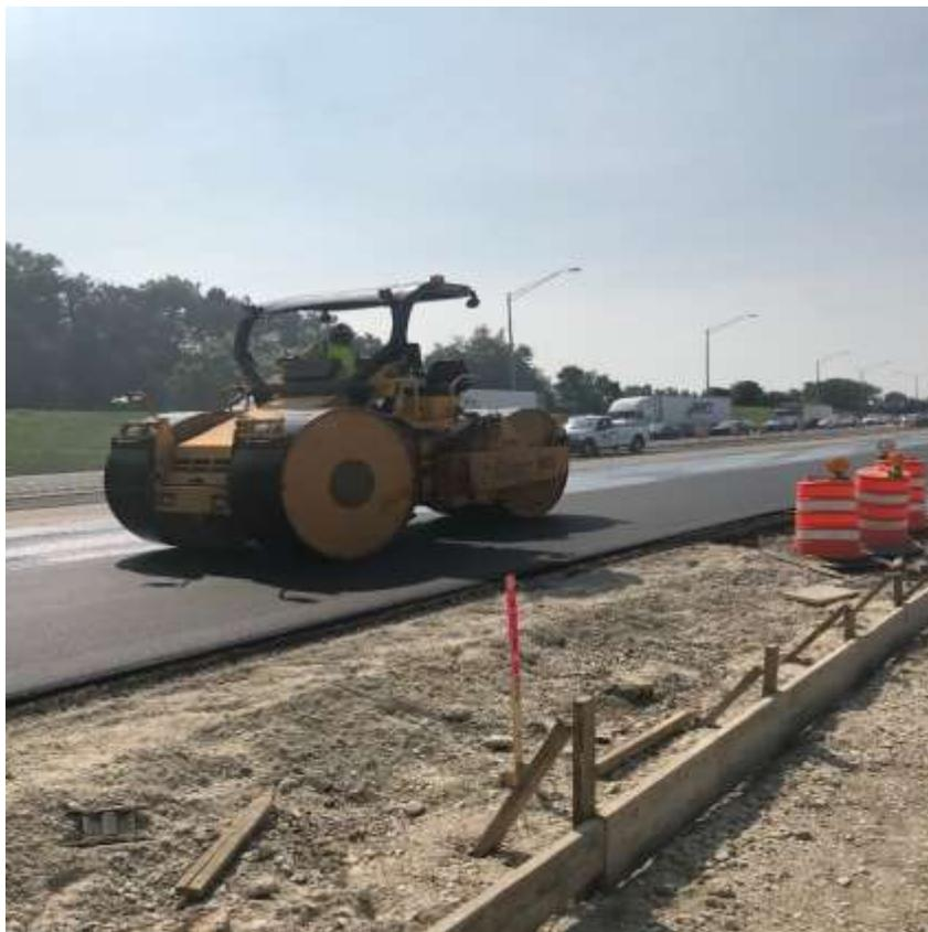
**Figure 5. Rolling over asphalt concrete.**
