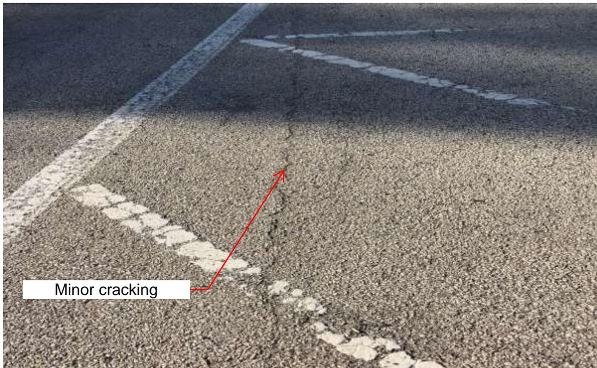
**Figure 7. Minor longitudinal crack.**
