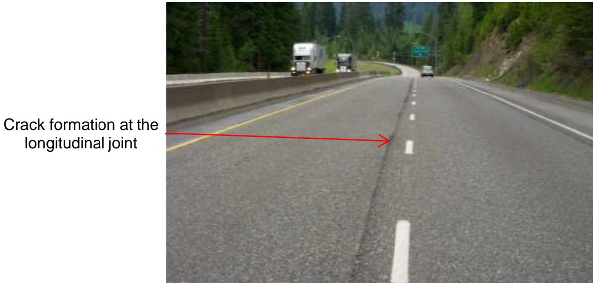
**Figure 8. Moderate longitudinal joint crack. (Pavement Interactive)**
