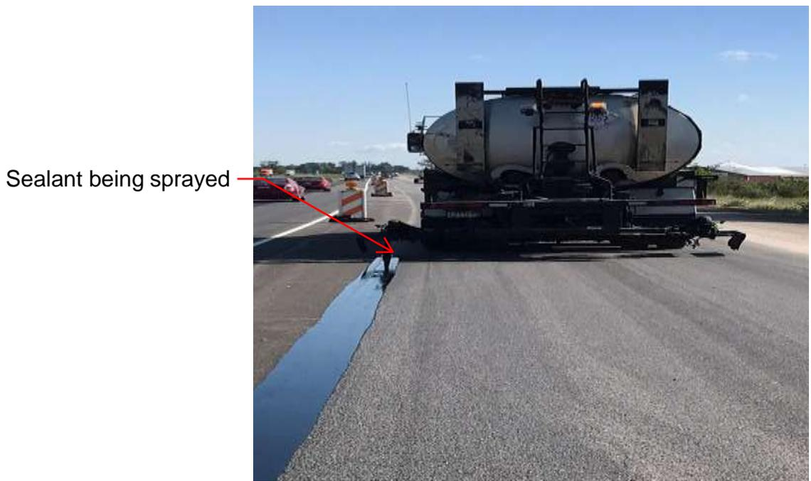
**Figure 11. Longitudinal joint sealant being applied.**
