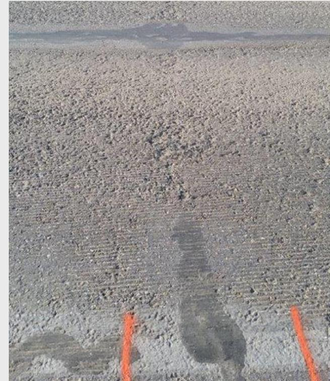
Non Working – Likely correctible by grinding or cold planing
