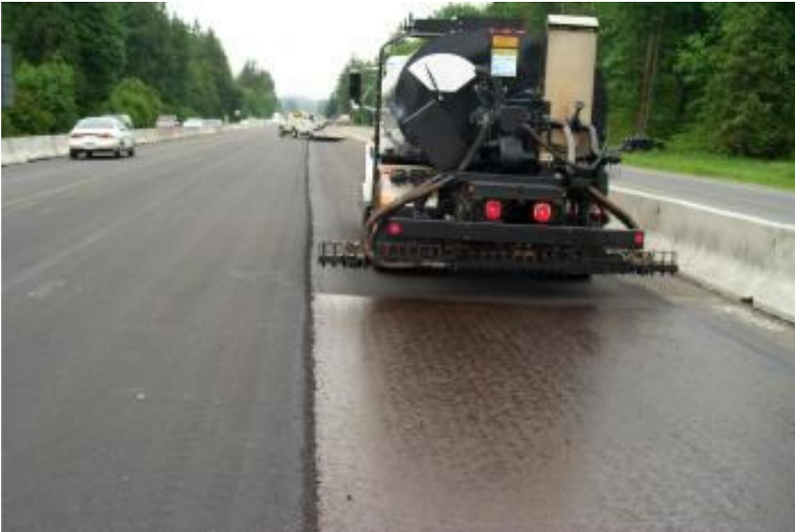
Figure 2. A truck applying the tack coat onto the pavement [2]
