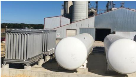
LNG Storage and Vaporization equipment to create Virtual Pipeline
