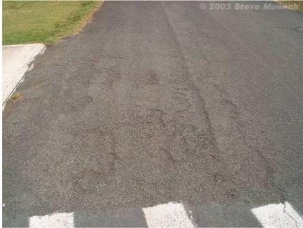
Raveling is the progressive disintegration of an HMA layer from the surface downward due to the dislodgement of aggregate particles. Raveling is described as losing debris on the pavement, rough, and collecting water in raveled locations. Raveling could be caused by aggregate segregation, inadequate compaction during construction, and asphalt binder aging (2, 3).
