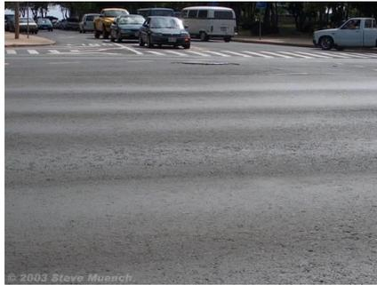
Rutting is a shear failure in the pavement. Due to traffic load, there are two types of rutting, one in asphalt concrete surface and another in subgrade soil.
