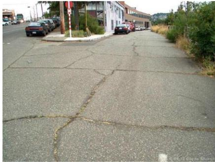
Joint cracking happens when asphalt concrete overlays rigid pavements over the underlying rigid pavement joints. Joint cracking is described as loose debris, moisture infiltration, and roughness. Joint cracking is caused by the movement of the rigid pavement slabs (3).
