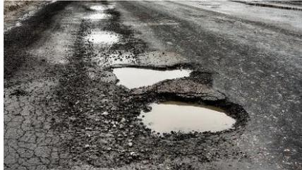
A Pothole is a bowl-shaped depression in the pavement surface that penetrates through multiple layers down to the base course. Potholes are generally the end result of cracks, including those listed above. Potholes are more prone to occur on roads with thin asphalt concrete surfaces. Potholes cause roughness and moisture infiltration, cause severe damage to the roads and vehicles (1).
