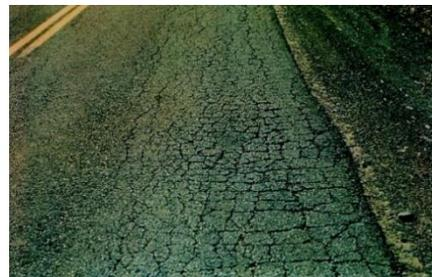
Fatigue cracks are a series of interconnected cracks caused by fatigue failure of the asphalt concrete under repeated traffic loading. Fatigue cracks allow moisture infiltration, decreasing the pavement load support and creating potholes (2).
