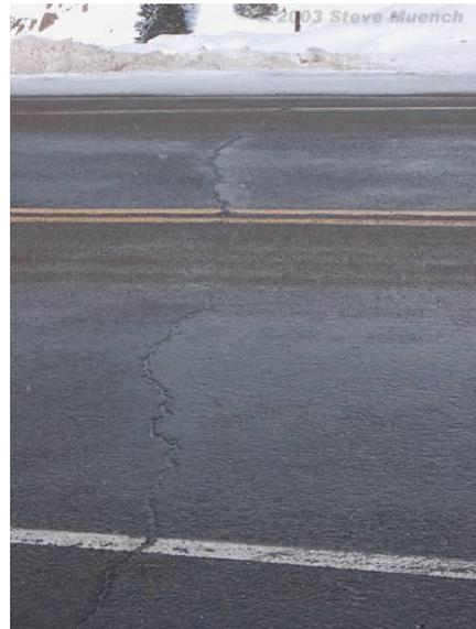
Thermal cracks happen when temperature differences within the pavement cause thermal stress and shrinkage, which cracks the pavement. These cracks are also known as transverse cracks (2, 5).
