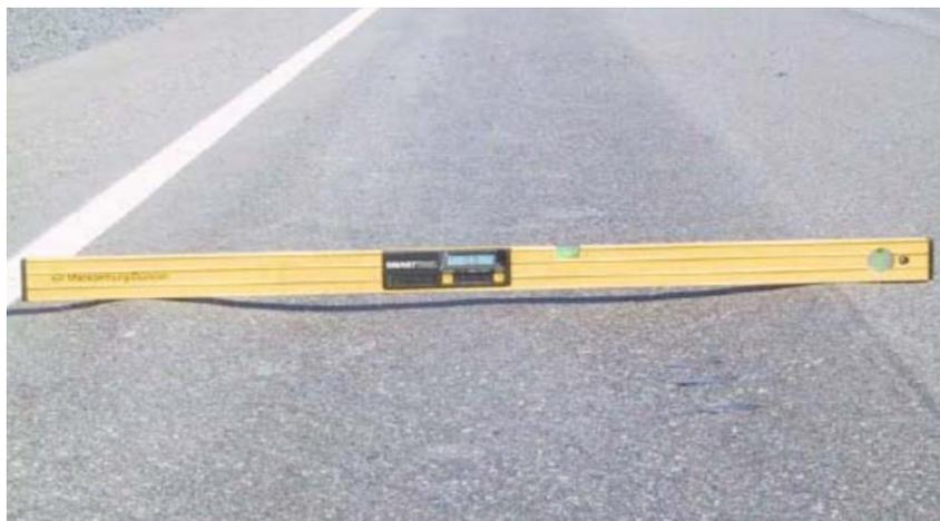
Figure 1. Typical Pavement Failure - Rutting
