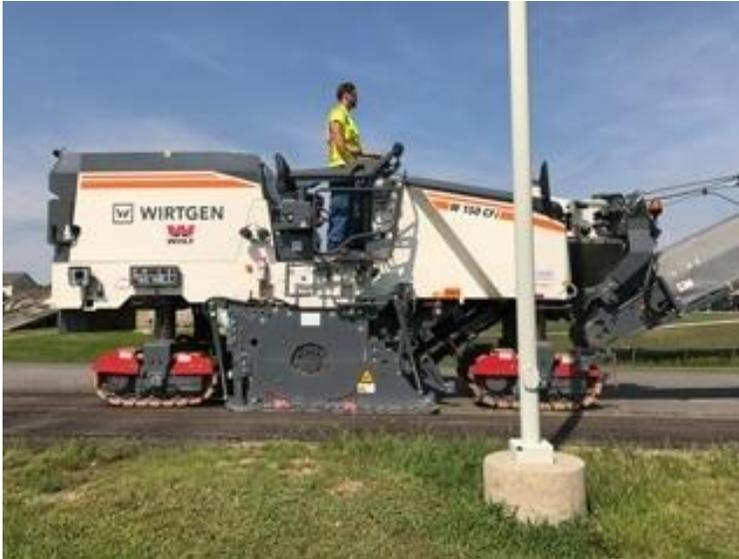
Figure 1) Roadway under milling process (8)
