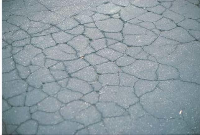
**Figure 4 Fatigue Cracking**
