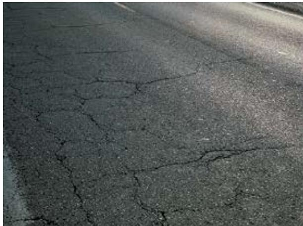
**Figure 1 Thermal Cracking**
