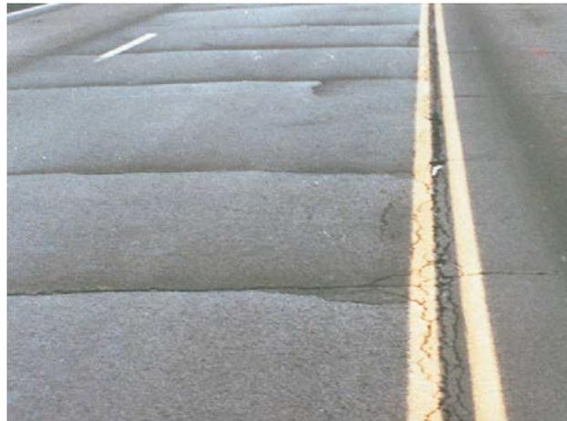
**Figure 3 Reflective Cracking**
