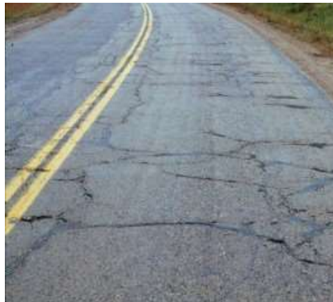
Figure 2 – Block Cracking
