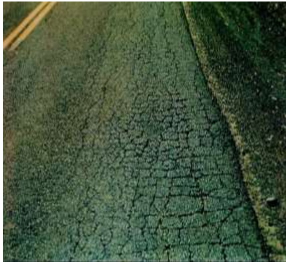
Figure 1 – Fatigue Cracking
