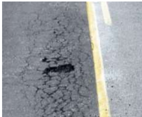
Figure 4 – Potholes
