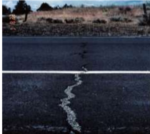
Figure 7 – Transverse Cracking
