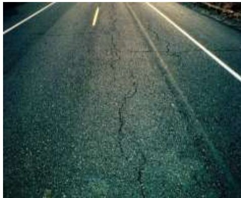
Figure 3 – Longitudinal Cracking
