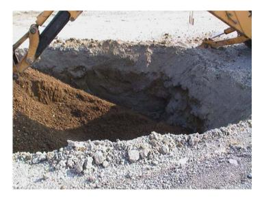
Figure 9. Excavation and replacement of soft grade and contaminated aggregate.
