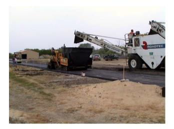
Figure 24. Paver and finish roller.
