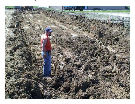
Figure 7. Undercutting at soft spot in Lane 1, aggregate lane.
