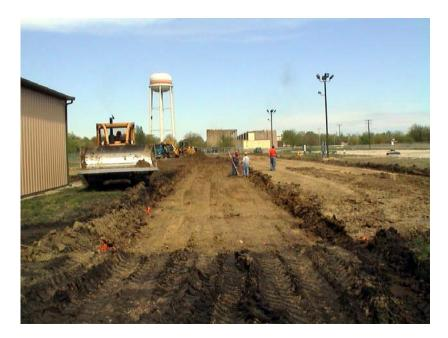
Figure 5. Lanes with topsoil removed.
