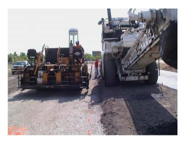
Figure 23. MTD on RAP center lane during paving.
