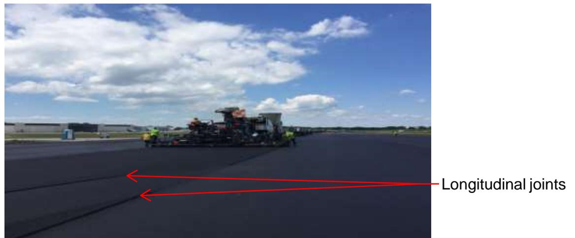
**Figure 1. Asphalt paving operation with a paver.**
