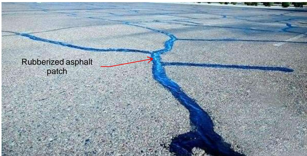
**Figure 10. Longitudinal joint repair using rubberized asphalt patch. (Keybot)**
