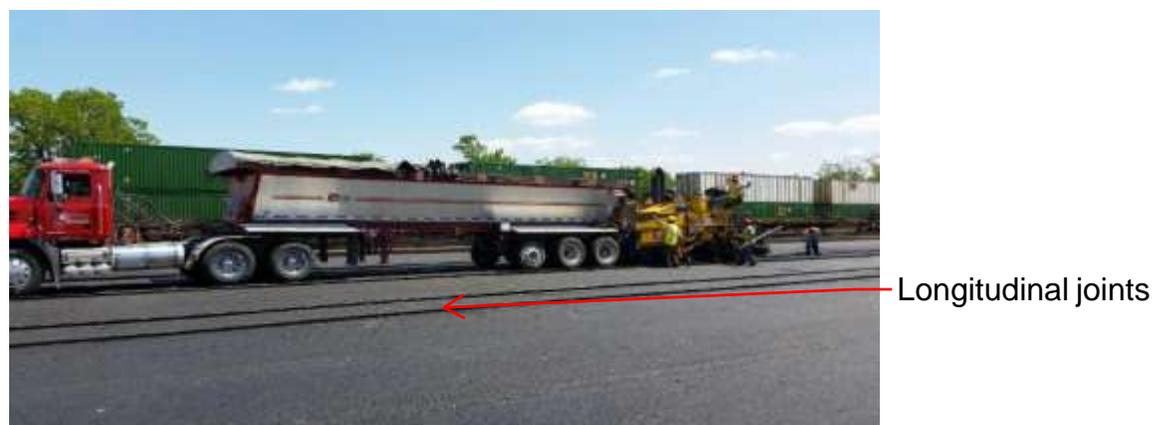
**Figure 2. Asphalt paving operation with a paver and flow boy trailer.**
