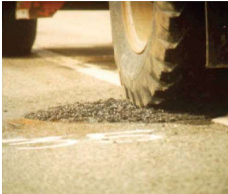
Figure 4: Demonstration of patching material being properly compacted with truck tires
