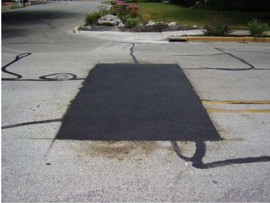
Figure 5: A finished semi-permanent patch (Photo NCHRP 2014)
