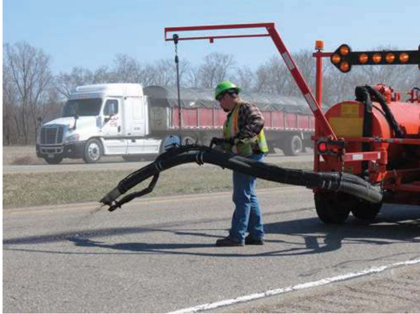
Figure 6: A trailer-mounted spray-injection patching operation (Photo NCHRP 2014)
