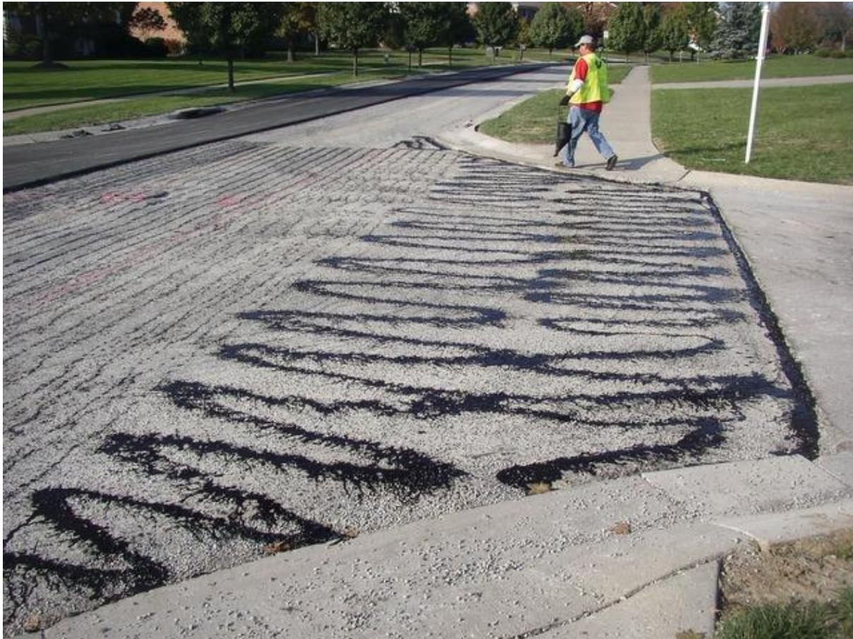
Figure 8. A lightly applied tack coat [8]
