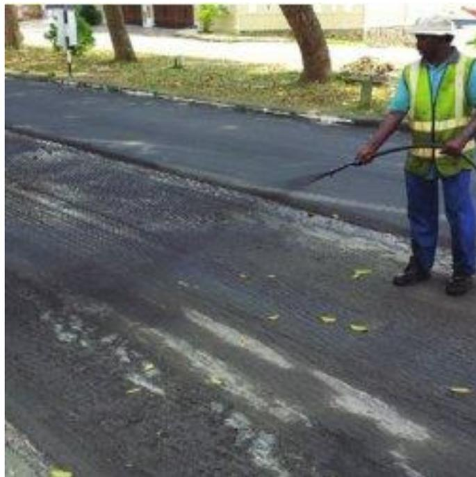
Figure 4. This is a man applying a tack coat with just a hose [4]
