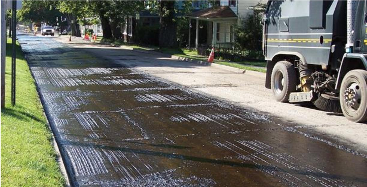
Figure 1. A tack coat applied to the first layer of pavement [1]
