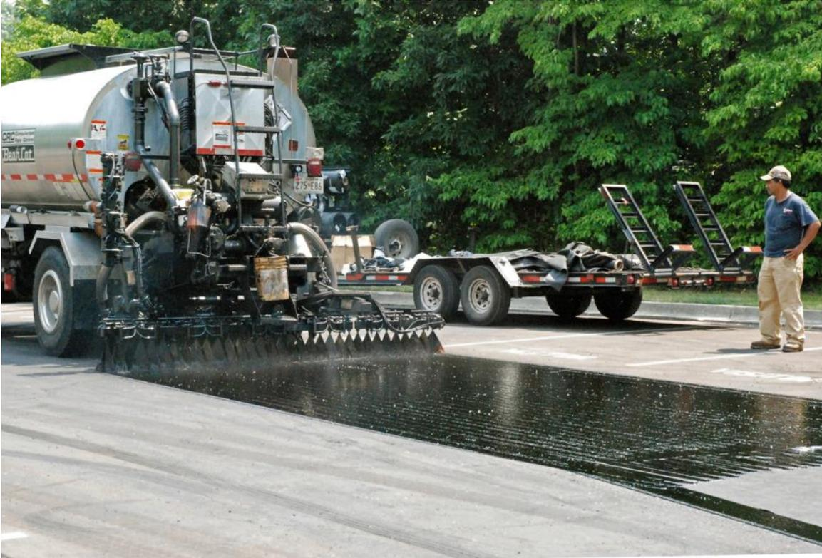
Figure 9. A heavily applied tack coat [9]
