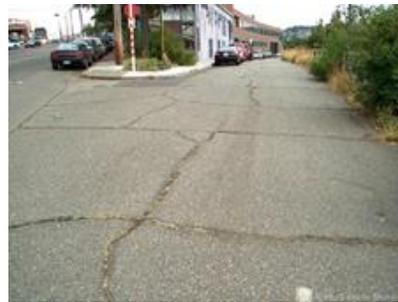
Fig. 1.5 – Joint Reflective Cracking, Pavement Tools Consortium
