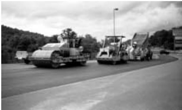
Rolldown of SMA mixtures is approximately one-half that of conventional HMA mixtures. While conventional HMA mixtures roll down approximately 20–25 percent of the lift thickness, SMA will normally roll down only 10–15 percent of the lift thickness.
