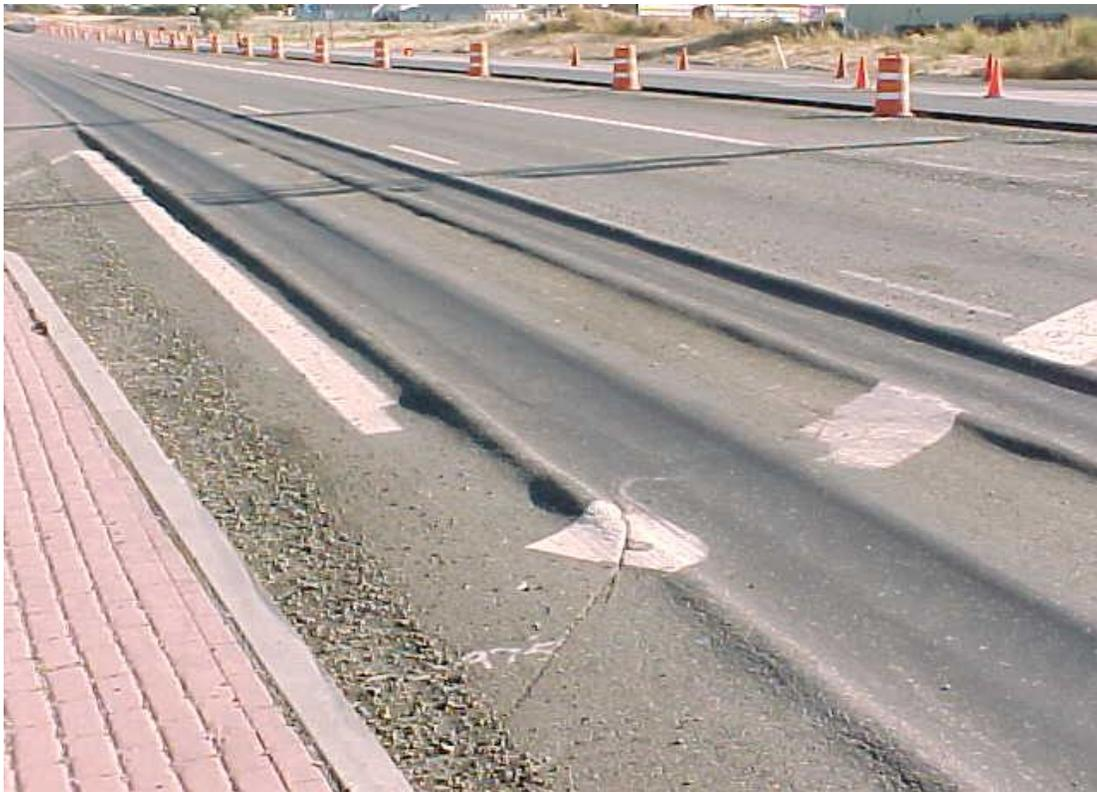
[Figure 2: Rutting of Asphalt roads](#)
