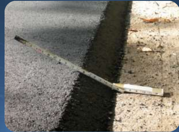
2010 Wisconsin Safety Edge Installation
