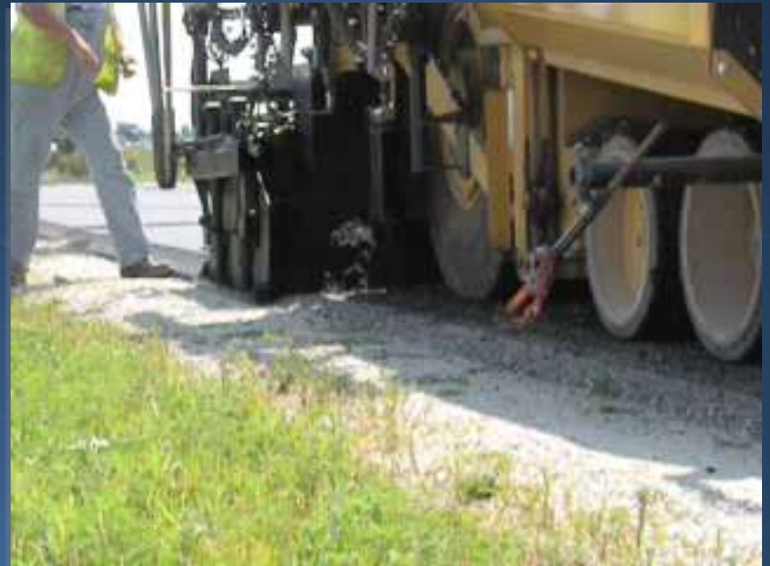
Paving with shoe
