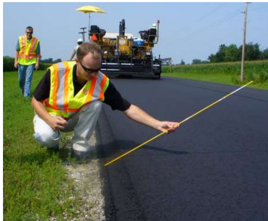
2010 Iowa Safety Edge Installation
