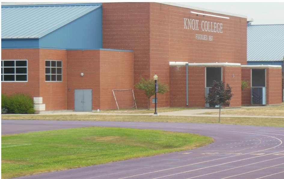
Running track with asphalt underlayment.
