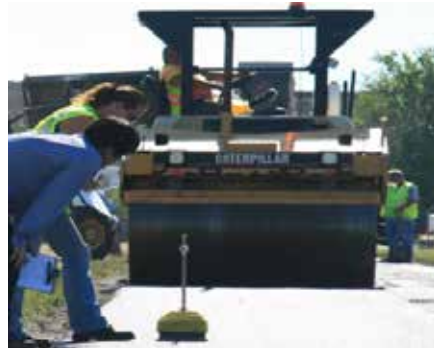
(g) Density measurement using nuclear gauge
