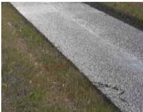
(c) Applying tack coat
