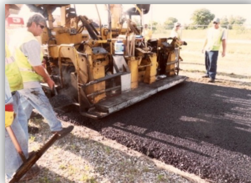
Figure D.6. Construction train (left) and paver-placed mixture (right).
