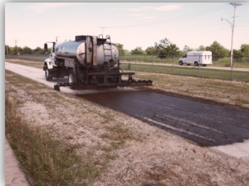
Figure D.5. Application of tack coat.
