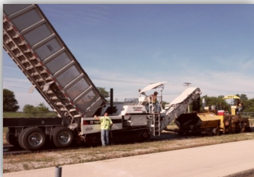
Figure D.6. Construction train (left) and paver-placed mixture (right).
