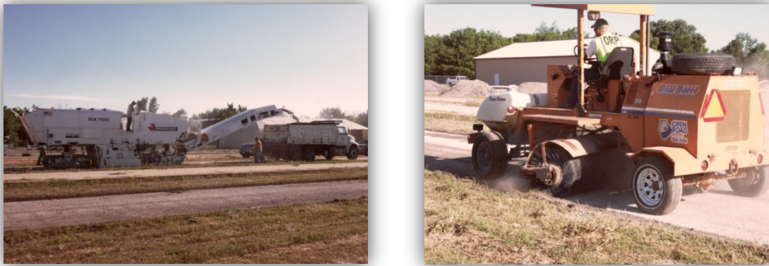
Figure D.4. Milling existing pavement.
