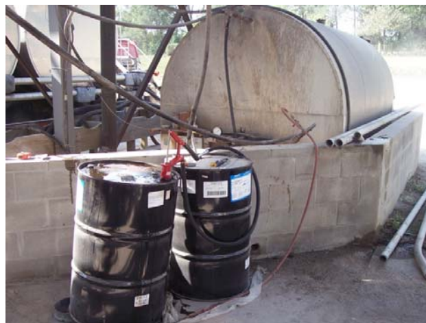
Figure 2.2 Injection of Evotherm™ 3G in the asphalt plant
