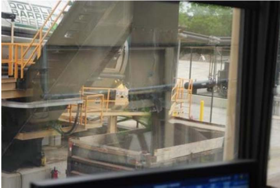
Figure 6.5 HMA mix discarded because it did not achieve target mix temperature.
