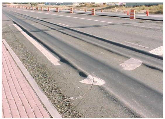
Figure 2: Rutting of Asphalt roads
