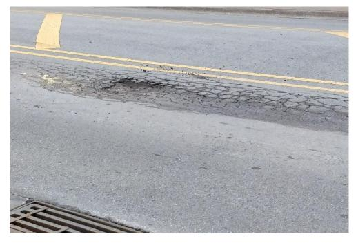
Figure 10: Potholes were formed in front of the ENGR Building, SIUC
