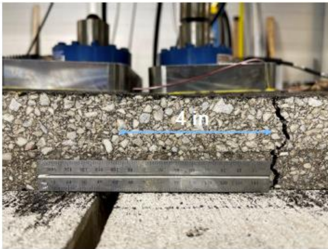
A single well-defined crack on edge cross section
