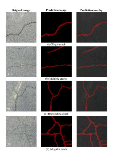
Figure 7. shows test results of four types of cracks in asphalt pavement (Ji et al., 2020).
