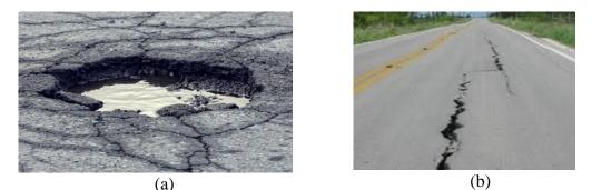
Figure 1. (a) A typical pothole and (b) Longitudinal cracks.
