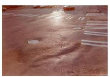
Shoving is a form of plastic movement, a wave (shoving) across the pavement surfaces. This distress usually occurs where traffic starts and stops. Shoving is described as roughness, unevenness, and irregular surface (3).
