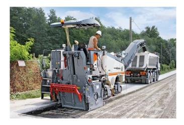
Figure 1: Milling Machine [1]
