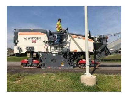
Figure 1) Roadway under milling process (8)
