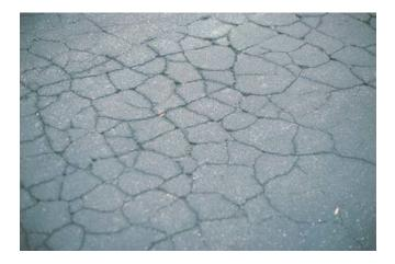
Figure 4 Fatigue Cracking
