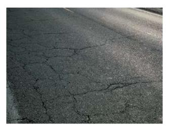
Figure 1 Thermal Cracking
