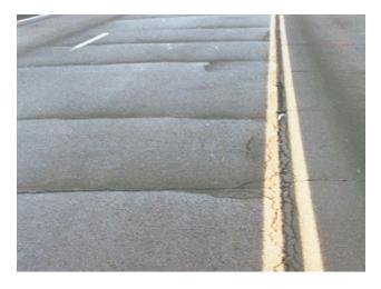
Figure 3 Reflective Cracking
