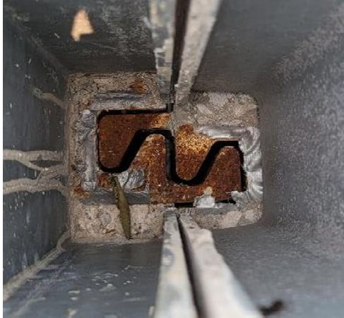
Concrete barrier locking mechanism connecting wall sections
